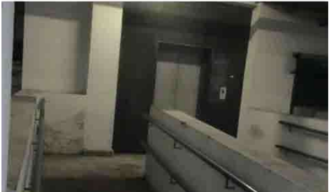
Ramp for disabled leading to Lift
